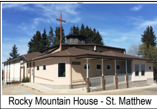
Rocky Mountain House - St. Matthew
